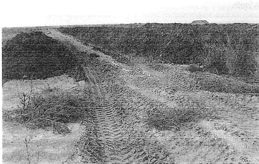
Photo 7. Completed windrows (photo by Ken Powell)
